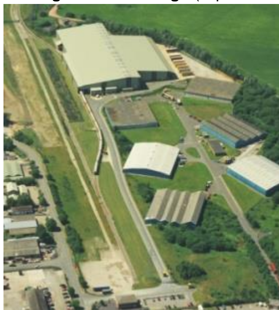
Figure 4: Waste Transfer Station at Knowsley Industrial Park with Rail Freight Terminal integrated into design (expected to be operational 2016)
